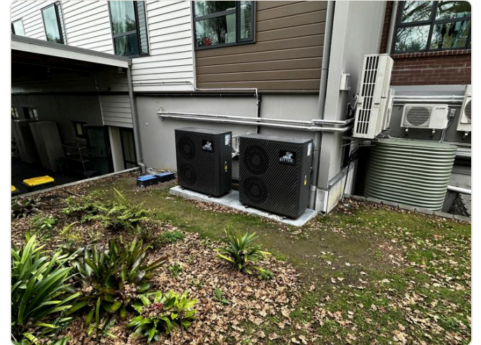
Two of the R290 units at one of the sites. Photo from the published project page.
